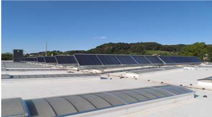
Figure 14. 276.64 kW th solar thermal plant for machinery and equipment industry in Switzerland (INTEC, 2015)
